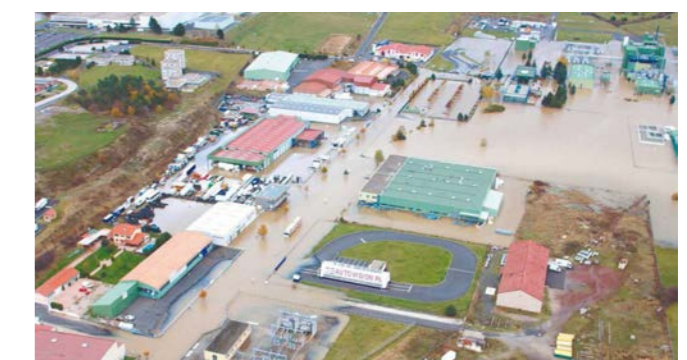
Figure 2: The affected site (Source: ARIA No. 35426)
