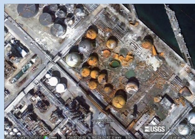
Figure 4: The LPG tank farm at the Chiba refinery after the earthquake-triggered fires and explosions (2012 Google, ZENRIN)
